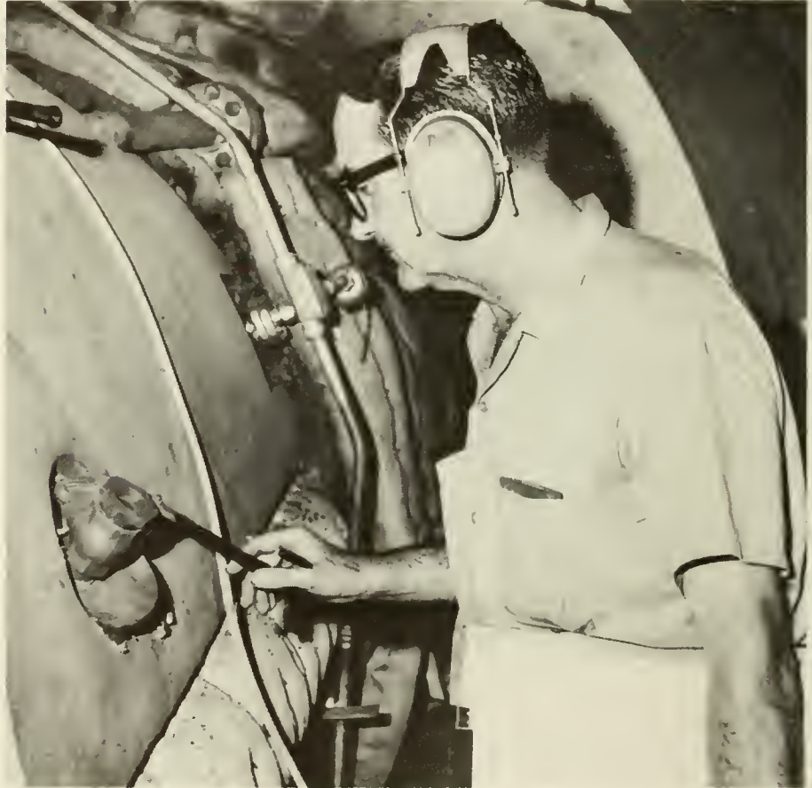
Ear muffs protect the hearing of Robert J. Roy, shift engineer on watch at the Miraflores Substation, shown checking one of the gas turbo-generators by making a flame inspection. Roy is inside the protective aluminum covering of the generator standing next to the generator itself. The asbestos padding over the turbine is a protection against heat.
